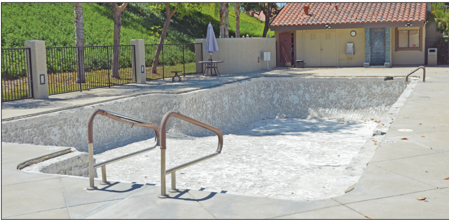
Pool 2 in June after being drained
