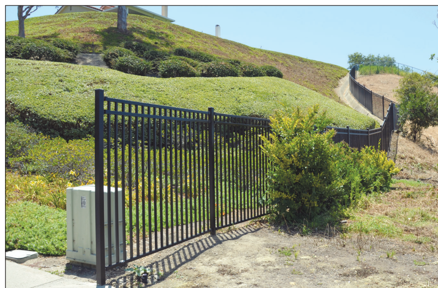
Replaced fencing by Gate 1
