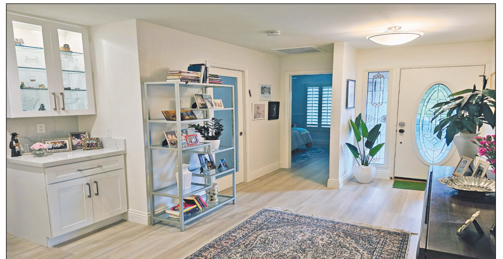
Hallway showing where closet was removed and cabinets installed
